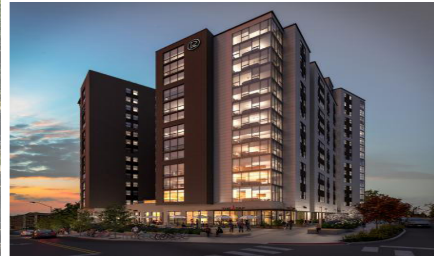
Facing Southeast Corner of State Street & Chauncey Avenue
