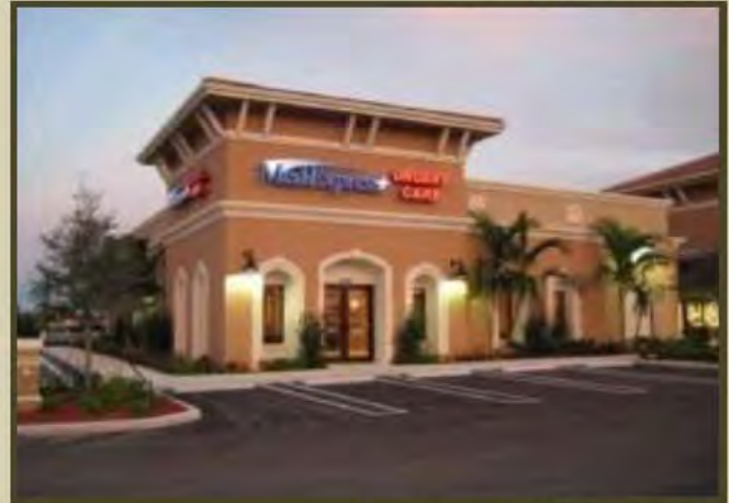
Free Standing Building (Florida)
