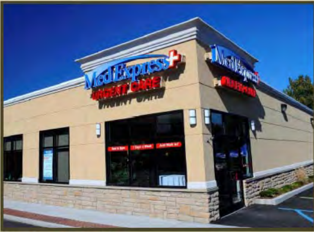
Free Standing Building
